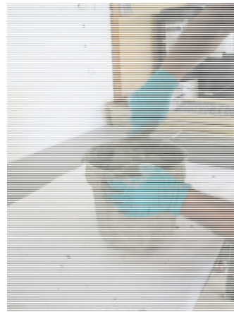
2. Thoroughly remix the mortar by hand methods.
